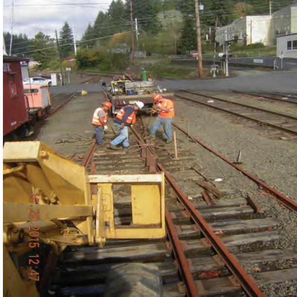
Conductor Tom, mounts flag on newly installed ground throw switch. Metal flag and post made by Mark Seibert in his shop.
